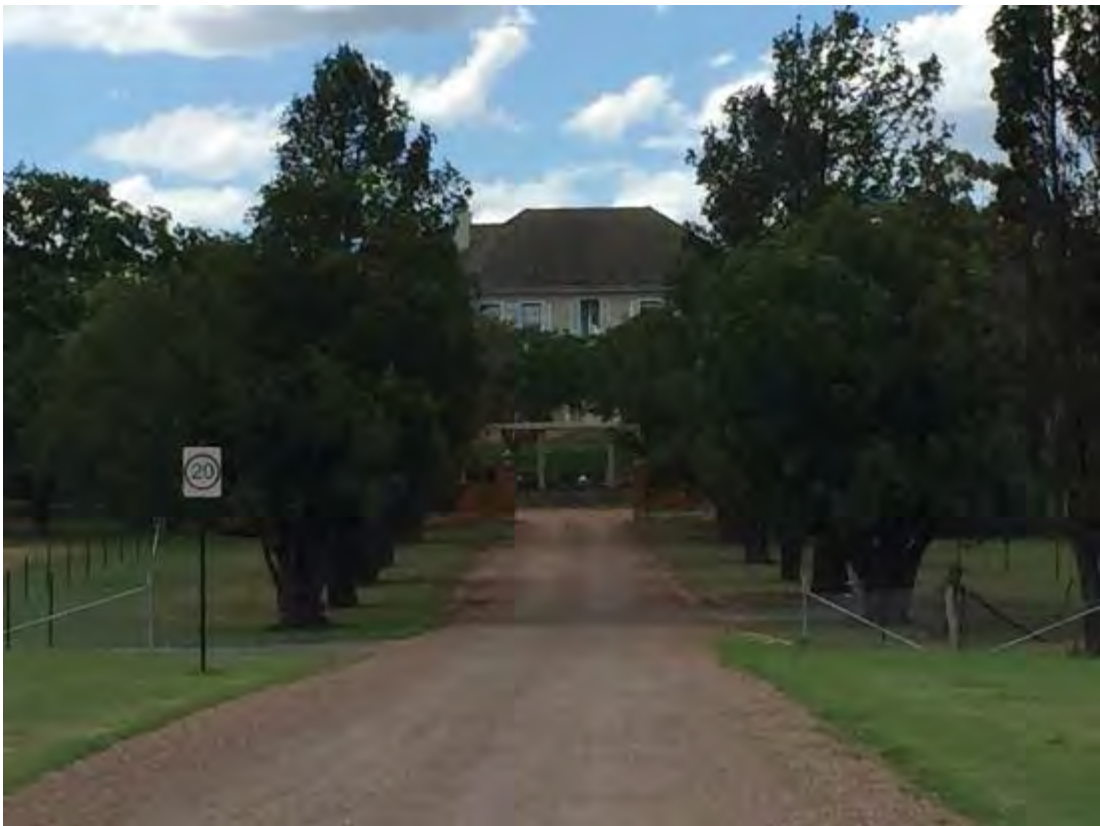
Figure 48: Zoomed in to the view of the Oran Park House formal entry. TTA Oct 2017
