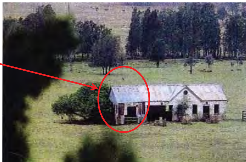
Figure 141: Coach House in 1992 showing the building was altered to a single storey structure with large openings and the stables are no longer extant. Belle – Design & Decoration, June/July 1992, pg.44.
