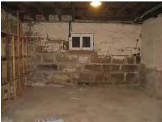
Figure 76: Cellar, Basement level, looking west. TTA 2013
