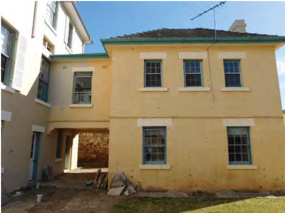
Figure 65: East elevation of the c1865 annex showing the link to the house built by Robbins. TTA 2013
