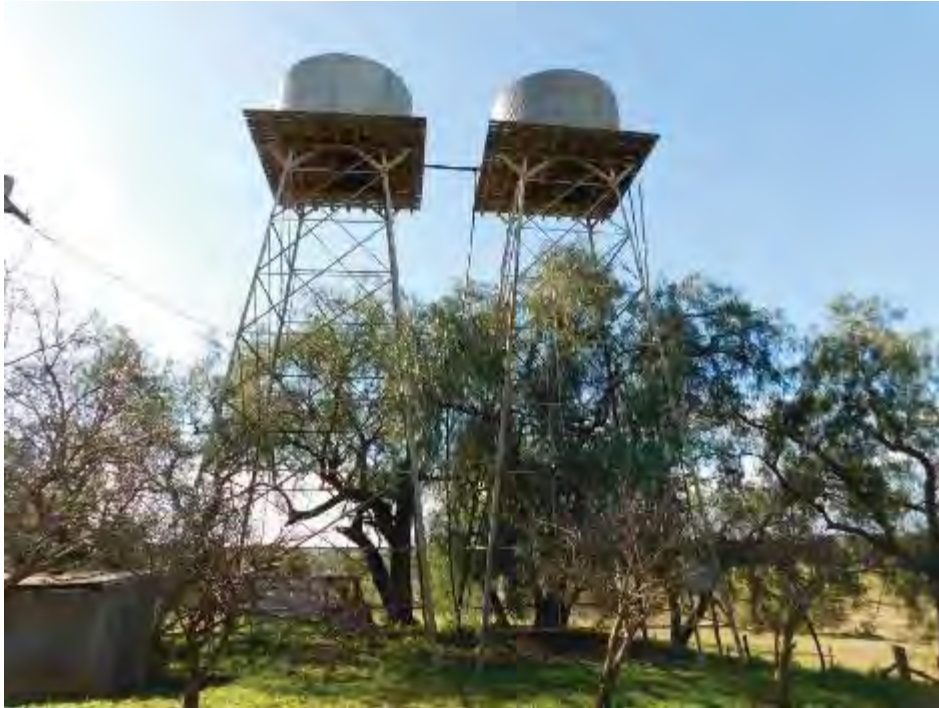
Figure 94: Water tanks looking north. TTA 2013
