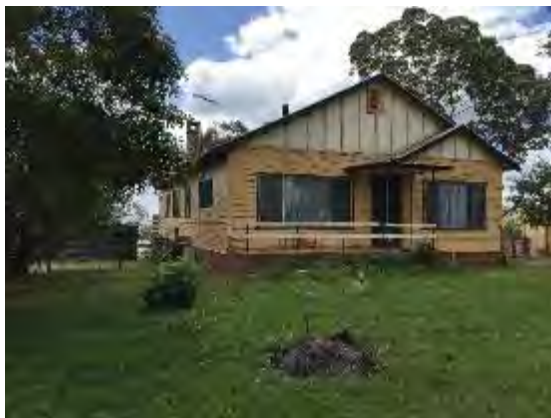
Figure 85: Caretaker's House, south and west elevations. TTA Nov 2017
