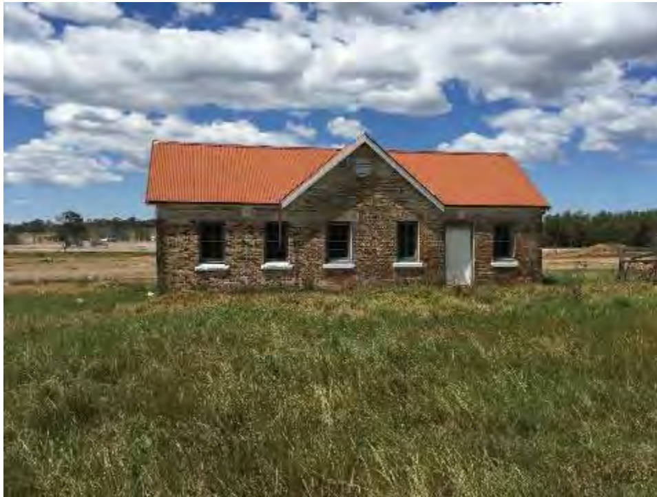
Figure 81: Coach House, west elevation. TTA Oct 2017
