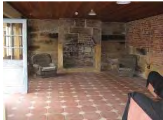
Figure 77: Former Garage (Girl's Dormitory), Basement level, looking east. TTA 2013
