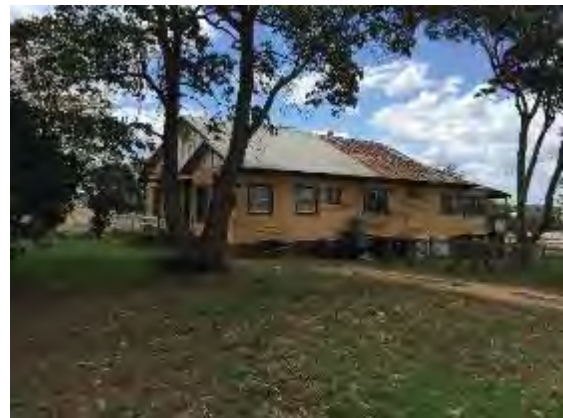
Figure 86: Caretaker's House, south and east elevations. TTA Nov 2017
