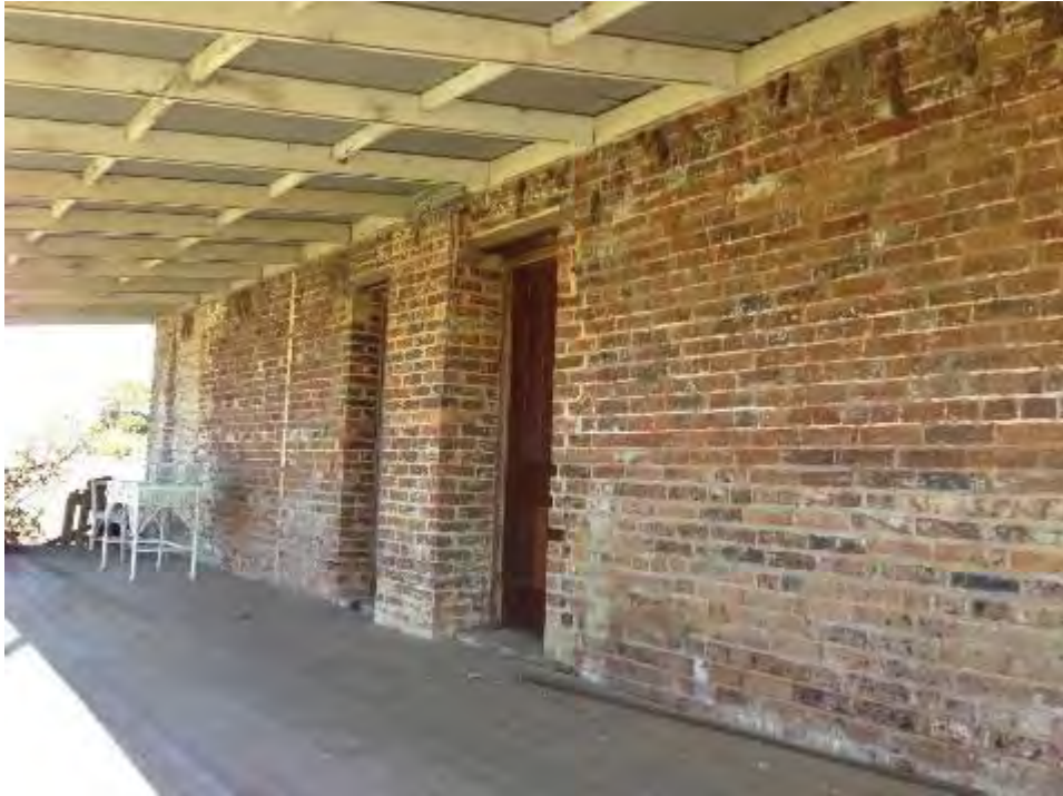
Figure 83: Coach House, verandah on the east elevation. TTA 2013
