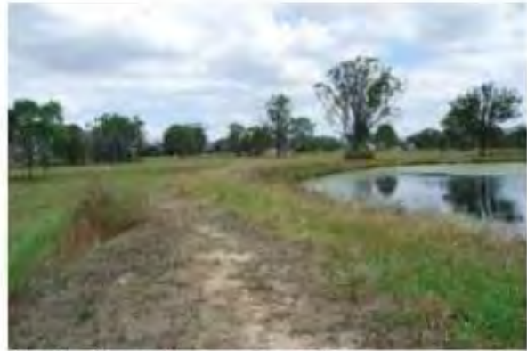
Plate 4. View south across dam wall
