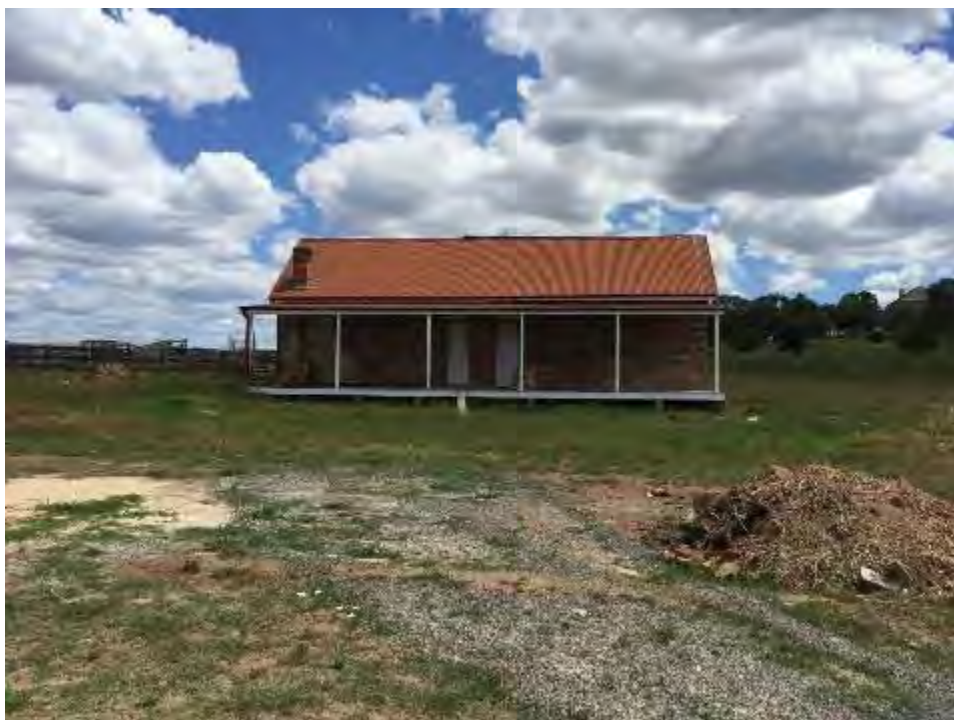
Figure 82: Coach House east elevation. Note Oran Park House to the right of frame. TTA Oct 2017
