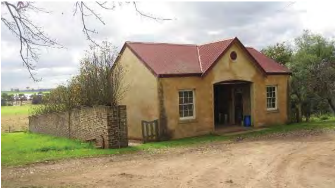
Figure 84: Garden Equipment Store, south and west elevations. TTA 2013
