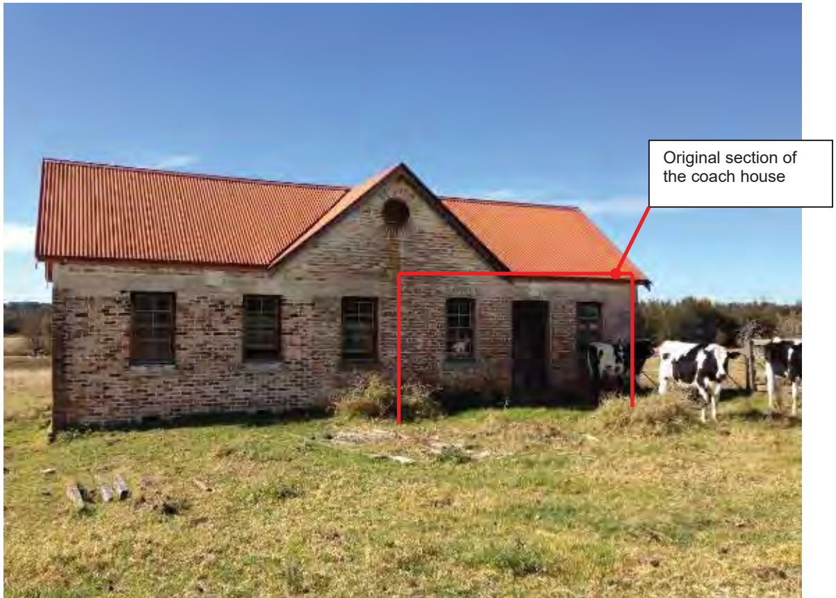
Figure 143: This images shows the original section on the west elevation of the coach house. Other openings have been reworked and the north end of the building demolished. TTA 2013
