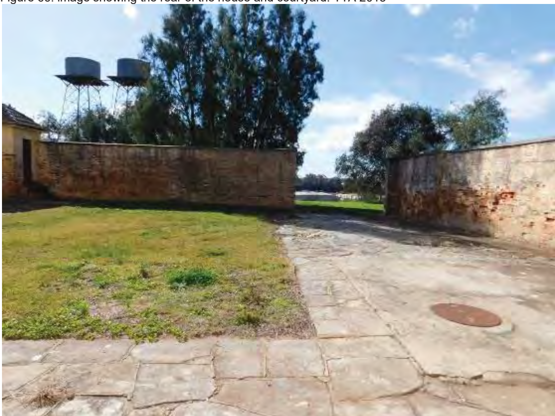
Figure 67: Rear of Oan Park House looking towards Water Tanks. TTA 2013
