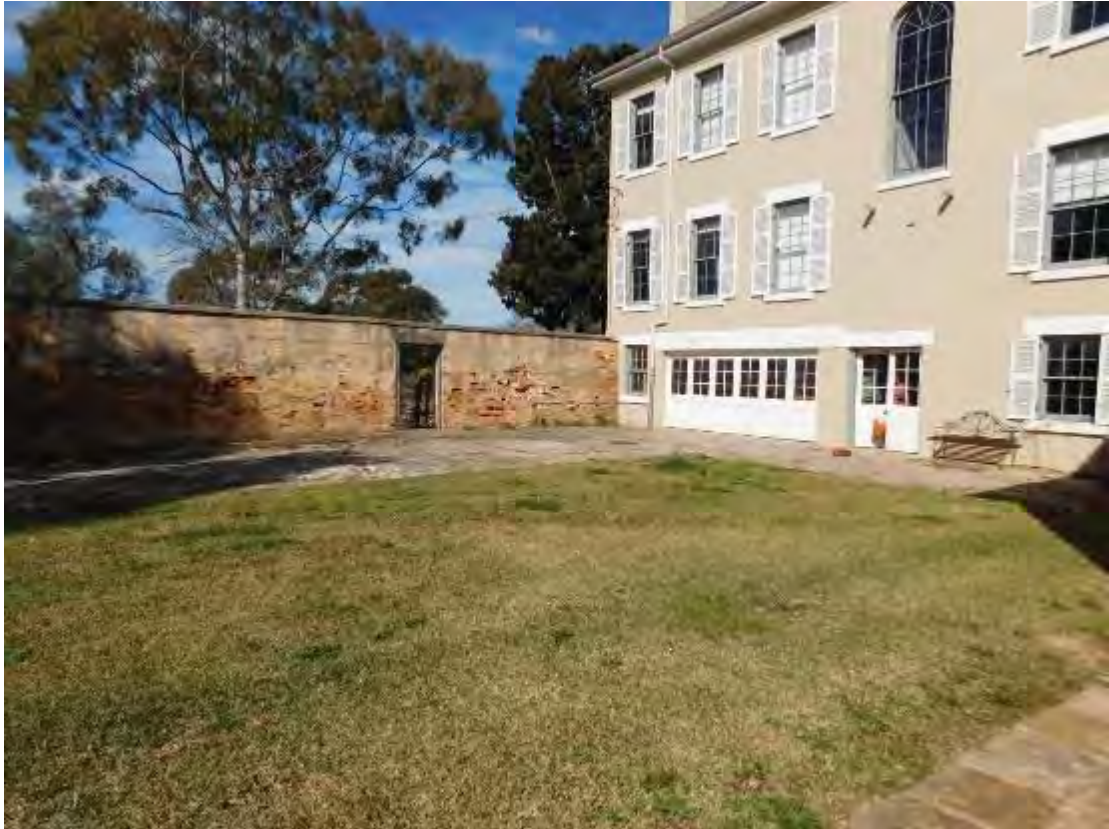
Figure 64: Rear (north) elevation of the house showing the generally symmetrical ground and first floors and the basement level. TTA 2013
